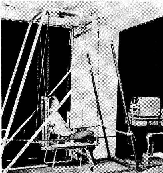
FIG. 1. General view of parallel swing apparatus. The oscilloscope providing the visual display (a circle shrinking as the swing moves forward and expanding as the swing moves back) is shown on the far right. The electrical pick-off from the swing controlling the display size is at the top of the structure on the right of the photograph. The horizontal ropes at hand level were not used in this experiment but were held by *S* to give proprioceptive information of movement in a later experiment.
